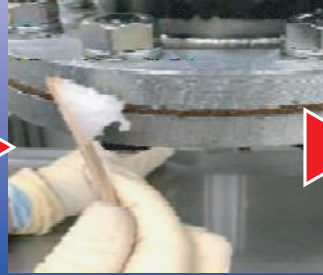
② Apply on leakage area
