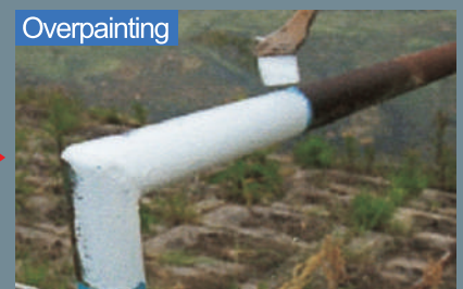
After drying, overpaint with general paint.
