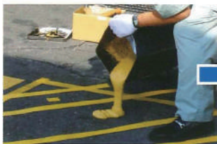
Drop the mixed non-slip coat directly to the painting surface
