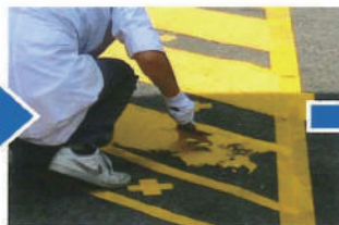
Spread to a uniform thickness around 1~2mm by rubber spatula
