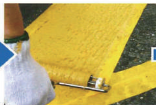
Use the special made roller for rough-patterning.
