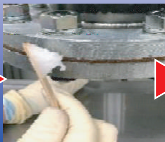
② Apply on leakage area
