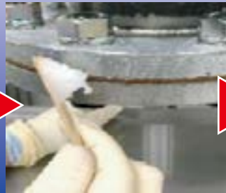
② Apply on leakage area
