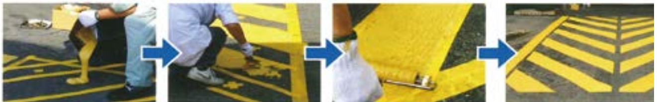
1.Drop the mixed non-slip coat directly to the painting surface
