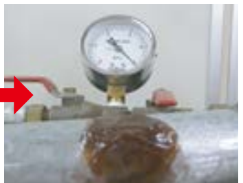
Curing is completed after return to natural temperature naturally.
