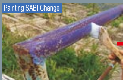
Apply SABI Change after the surface preparation (SP3).
